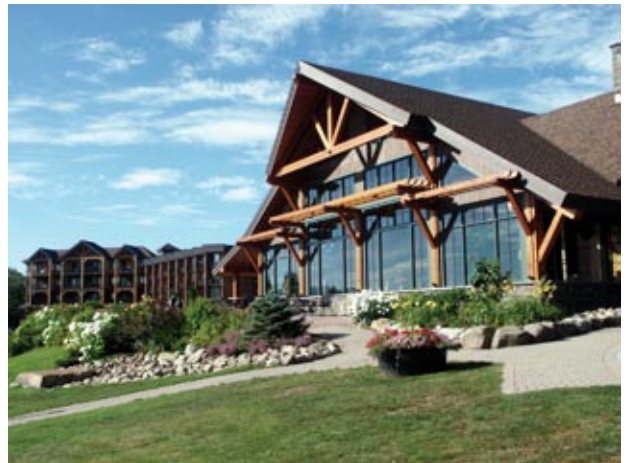
Great Room Lobby exterior
